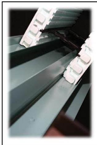
poured into the cavity. Upon curing, the insulated panels remain as an outer shell of the concrete wall on both the exterior and interior. In addition to superior structural strength, this construction method provides superior insulation, and in some residential projects means that no further insulation (such as blown fiberglass) is needed. ICFs are also green building products that contribute LEED points to projects, since they reduce energy costs.<sup>2</sup>
