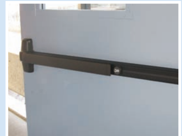
Von Duprin CD99 rim exit device used on doors leading outside incorporate cylinder dogging
