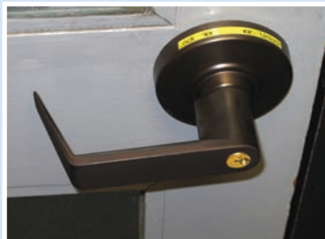
Classroom security function of Schlage lock provides a key lock inside the classroom so the teacher can remain inside during a lockdown situation.
