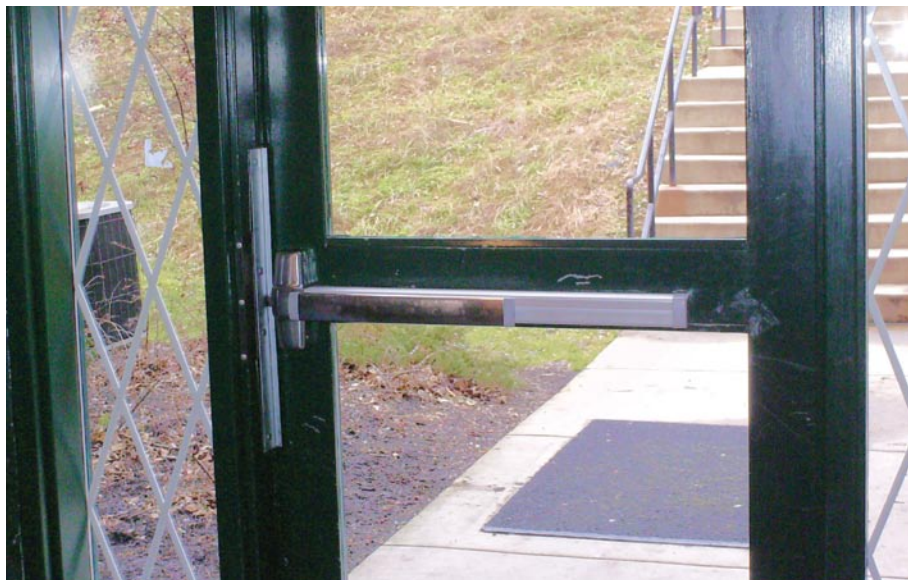
▲ Closeup shows a newly installed Von Duprin XP99 exit device on a door that is undergoing renovation. ▼ Von Duprin EL99XP exit device on this dormitory door incorporates electric latch retraction to provide access control. LCN door closer provides positive closing to ensure secure latching.
