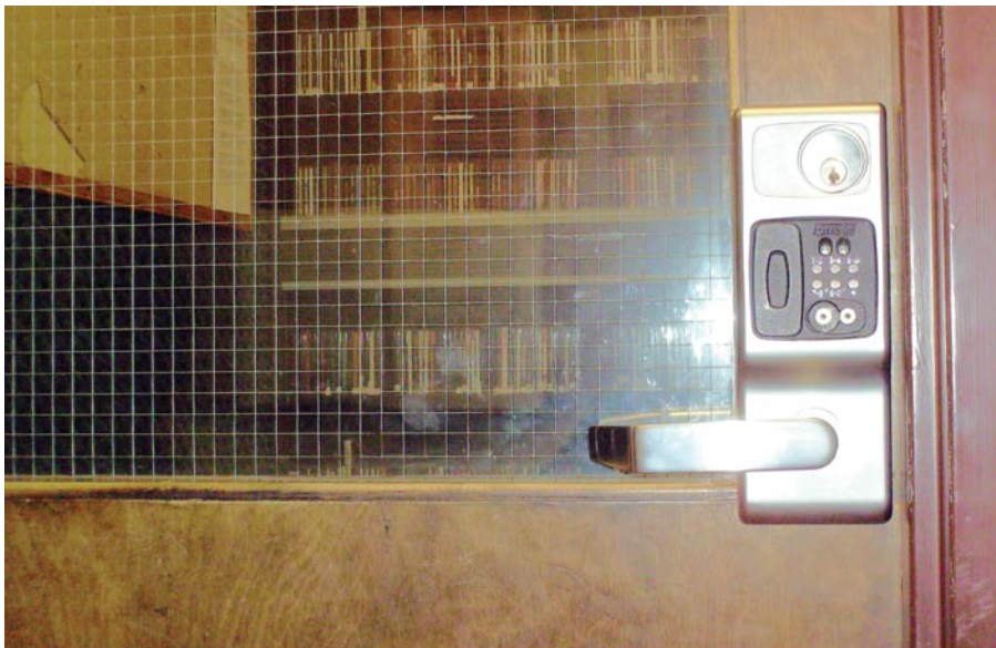
▼ Schlage CM lock incorporates proximity card reader to protect this laboratory on campus
