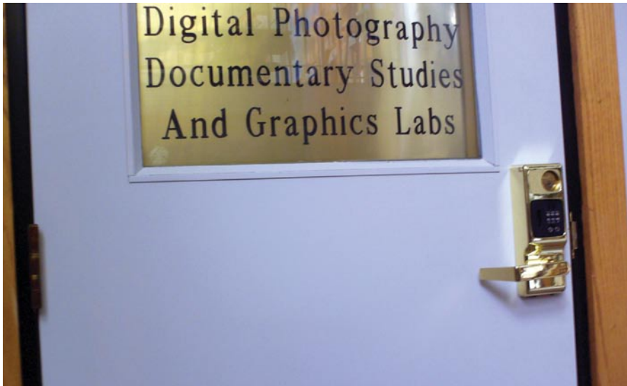
▲ Campus radio station is protected by a Schlage computer-managed (CM) standalone access control lock set.
