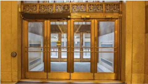
In order to meet accessibility standards, the two glass panels that previously separated the sets of three doors (original to the left) were moved to the edges and replaced by slightly narrower bronze flush panels.
