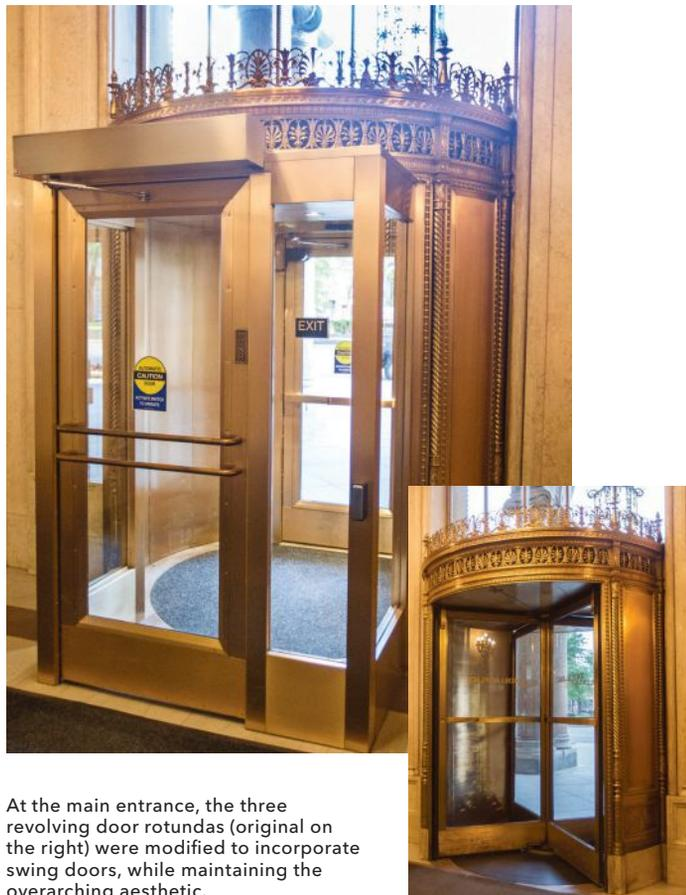
At the main entrance, the three revolving door rotundas (original on the right) were modified to incorporate swing doors, while maintaining the overarching aesthetic.
