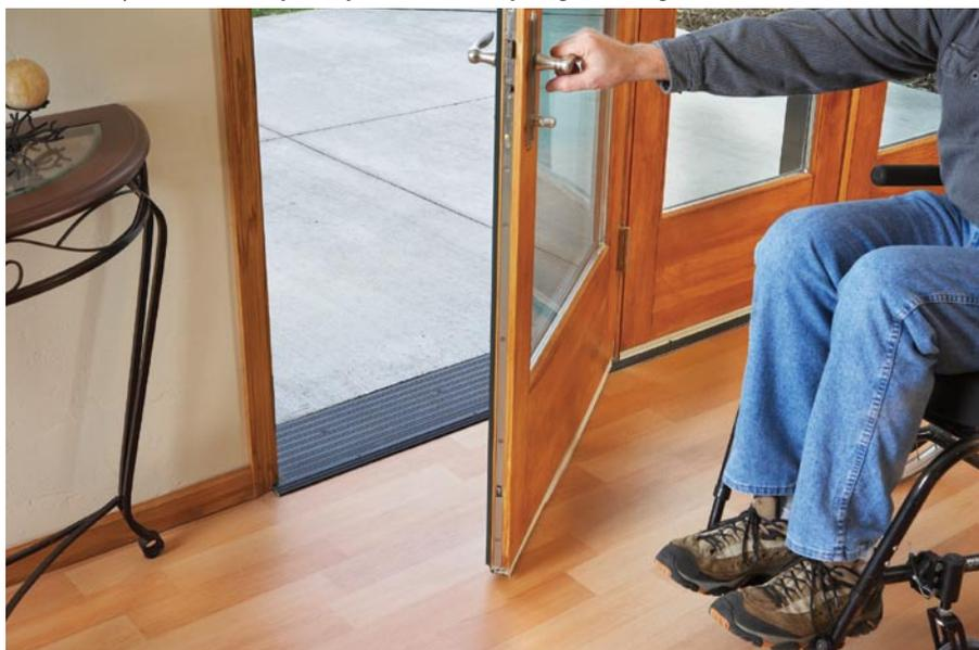
Kolbe's universal design exterior doors with flush-to-floor sills are engineered into the doorframes as integral components to ensure that the finished floors align with the thresholds.
