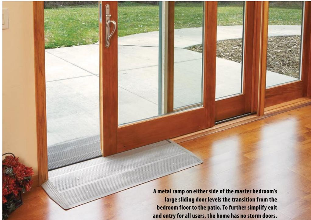
A metal ramp on either side of the master bedroom's large sliding door levels the transition from the bedroom floor to the patio. To further simplify exit and entry for all users, the home has no storm doors.
