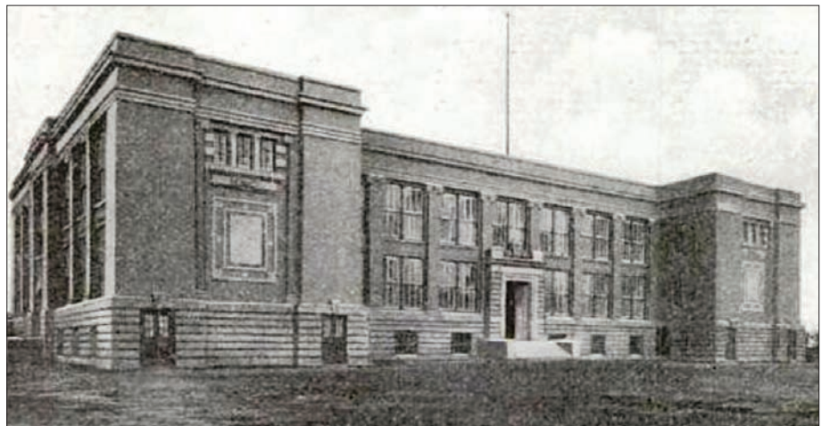
Collinwood Elementary School, built after the prior building burned down with massive loss of life. The "new" school gave every classroom direct access to the ground.
